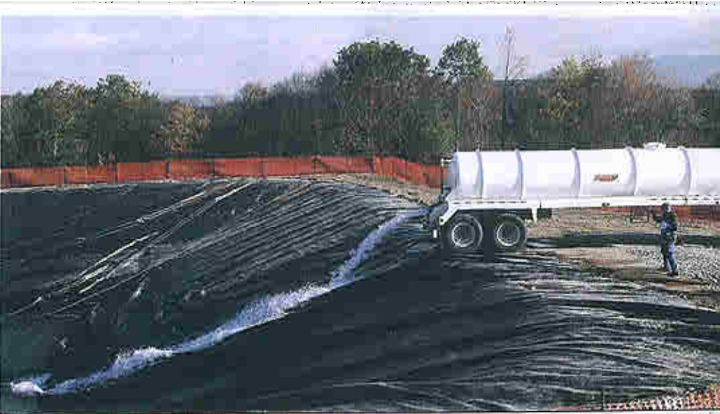
Left: More than two million gallons of water per well are injected to release natural gas from the shale formation. Disposal of the contaminated frac water poses environmental risks. Right: Wells are capped after drilling.
