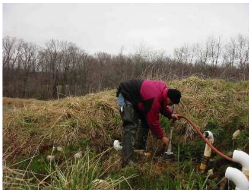
Tim Danehy, BioMost, Inc. backflushes treatment cell, which is needed every 2 years to maintain flow.
