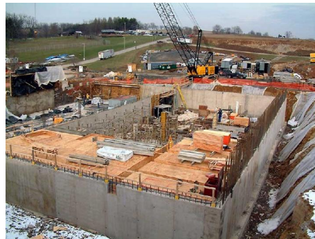
Advanced Water Treatment Building Under Construction
