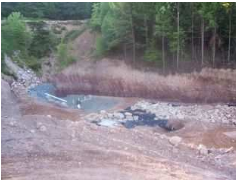
Mine Tunnel Discharge is redirected.
